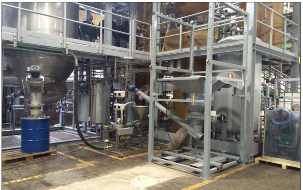
Dynasafe Workshop in Germany—building the off-gas treatment unit
